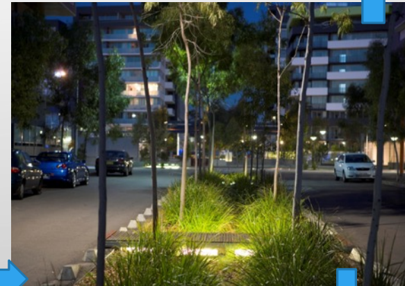
Urban runoff Biofilter
